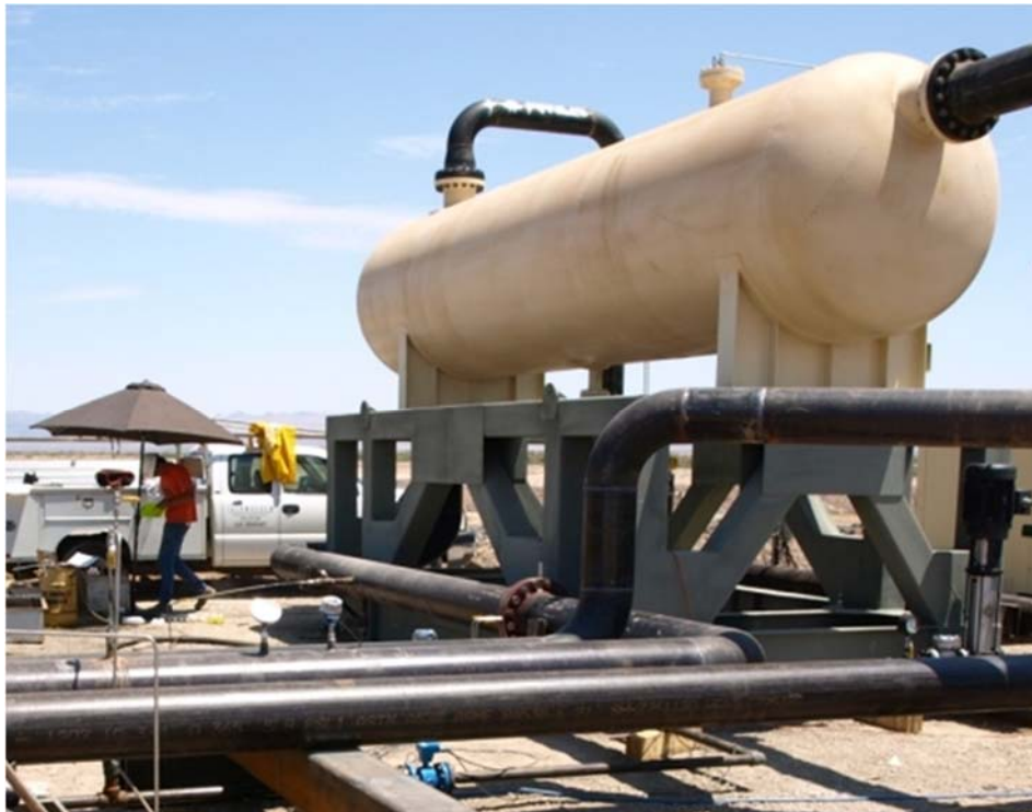
Figure 2. Production Test Separator
